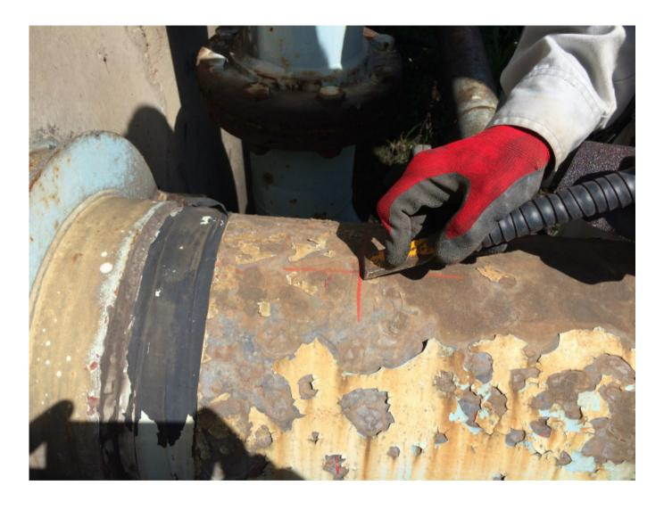
The points marked need to be scratched by a tool or/and sand paper. We will not use grinding wheel or other tools that will spark.
