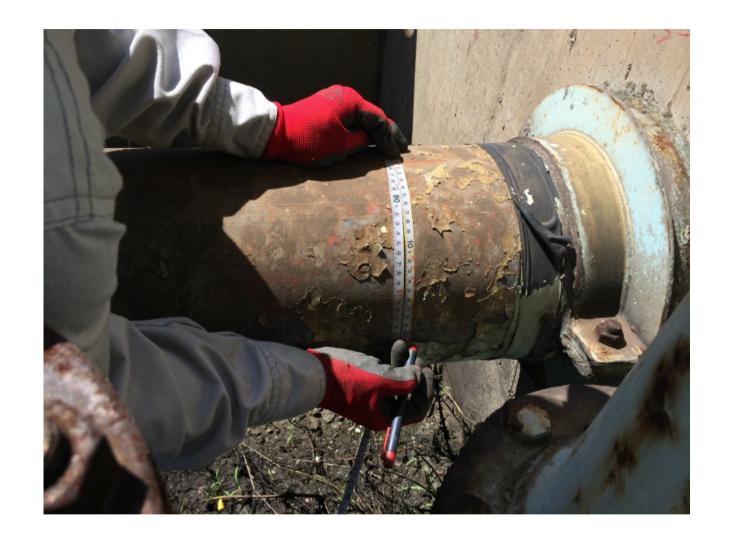
To mark the points for electrode and sensor pins.
